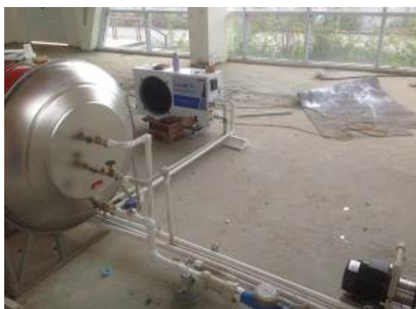
Figure 10 – Installation of Solar Hot Water Plumbing System Model
