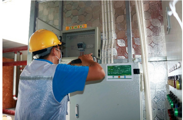
Figure 19 – Installation of the M&V system at CUWC
